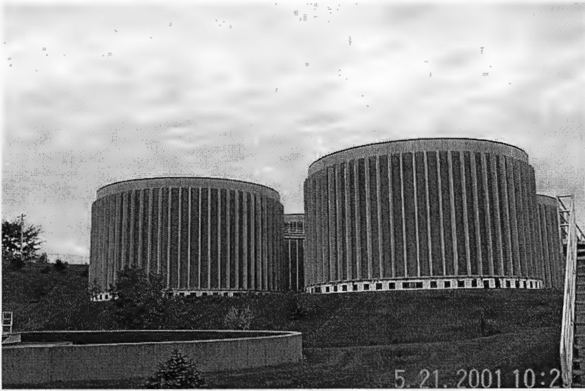
Figure A1. AWPCF trickling filters: NTFs are in the foreground and TFs are in the background.
